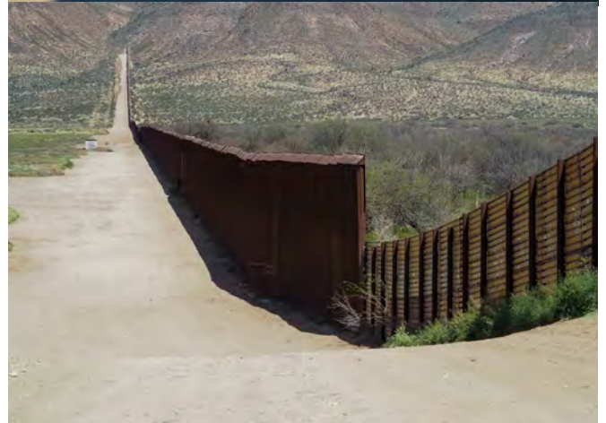
Border fence near Jacumba in eastern San Diego County. The image from 2002 (above) shows the 8-foot fence constructed from surplus landing mats and then a vehicle barrier in the valley bottom. The 2017 image (below) shows how the vehicle barrier was replaced with a pedestrian fence approximately 20 feet in height that also includes gates that open to accommodate stormwater flow and decrease flooding impacts.
