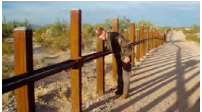
This steel fence is designed to stop car and truck traffic that used to drive from Mexico, through the wilderness of Organ Pipe Cactus National Monument, to enter into the United States illegally. This type of barrier does not impede wildlife following traditional migration corridors.
