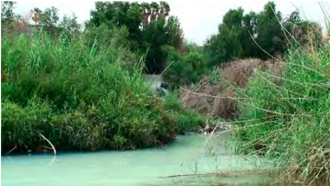
A small outfall emanating from a concrete structure draining into the Rio Grande.
