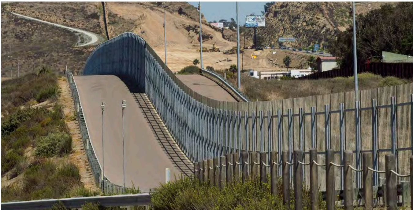
Border security infrastructure near Border Field State Park in San Diego County adjacent to the Pacific Ocean. The infrastructure includes the fence near the boundary, an access road, stadium lighting, a secondary fence and an additional road.
